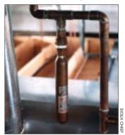
To prevent water hammer, install an arrestor near the fixture. It contains a bellows and spring to absorb some of the energy of the flowing water, but cannot become waterlogged the way an expansion chamber will.
