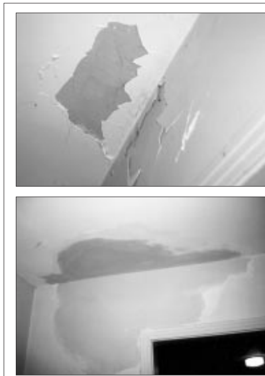
Repairing minor water damage. Water from a roof leak caused the top coat of plaster to separate from the base coat (above, left). To repair the area, the author scrapes away the loose top coat, leaving the base coat intact (above). Note the dark area in the inside corner; this is rust on the metal lath. The author then seals the area with a white-pigmented sealer and finishes with two coats of fast-setting joint compound (left).
