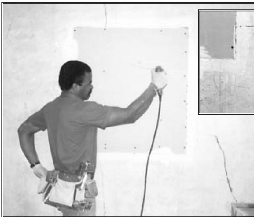
In a typical repair, the author removes a square area of deteriorated plaster, seals the raw plaster edges, then attaches a \frac{3}{8} -inch drywall patch. He reinforces a nearby crack with plaster washers (above) before taping and finishing the area with a fast-setting joint compound.
