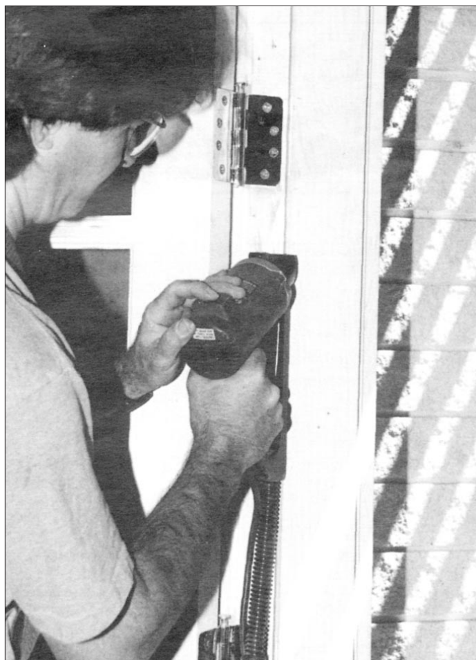
The V-shaped base of RCT's tool positions the bit to cut a simple kerf in the corner between the stop and jamb. The hose attaches to any standard vacuum cleaner inlet to help remove sawdust.
