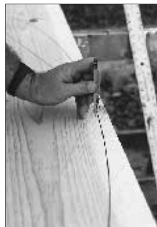
Figure 2. To draw an elliptical arch, the author first lays out the spring line and rise of the arch. He finds the focus points by pulling a tape from the top of the rise to the spring line and measuring one-half the length of the arch opening. He then stretches picture hanging wire from focus point to focus point, passing the wire over a temporary screw at the top of the rise (A). Finally, he removes the screw from the rise and scribes the ellipse with a pencil, pressing it firmly against the wire as he moves it from focus point to focus point (B).
