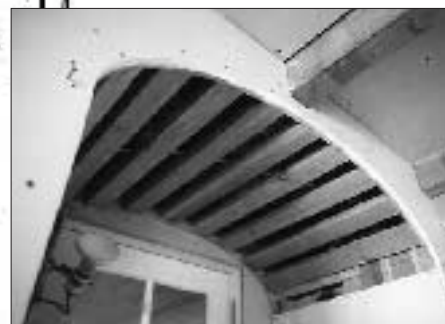
Figure 3. The author assembles the pine arch forms with 2x spacers. He positions the arch assembly tight to the header above, attaching it to 2x blocking nailed to the jack studs. Another option is to use long spacers as joists to make a vaulted arch (inset).
