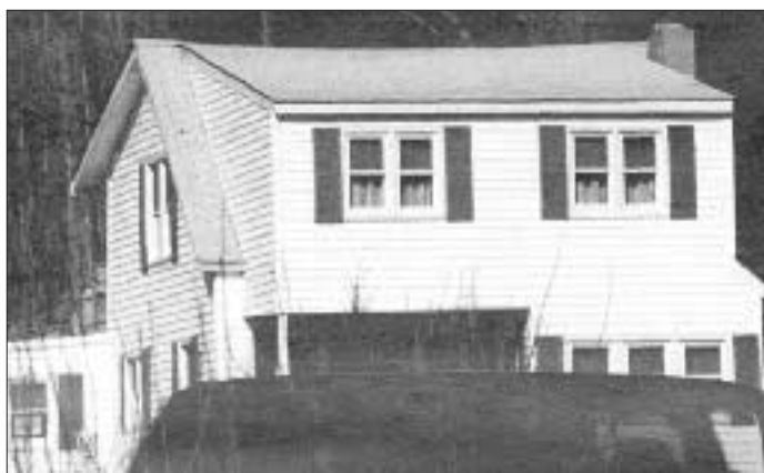
Shed dormers are often retrofitted in roofs where the framing is undersized. The result is a sagging ridgeline.
