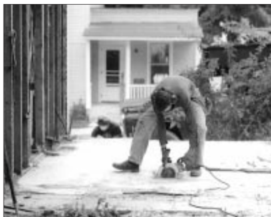
The chances of cutting a nail during this demolition project are high. When this happens change the blade immediately. If you don't, the blade will heat up and become ruined, and you risk a dangerous kickback.
