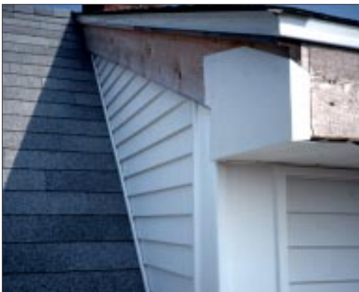
Figure 6. The aluminum rake returns (left) lap over the ends of the soffit and bend around the end grain of the wood rake and the back of the wood return. The aluminum rake and fascia then lap over the aluminum return (right).
