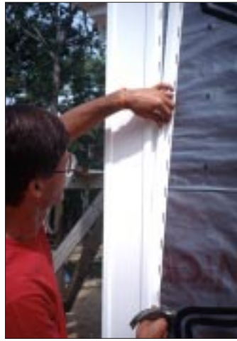
Figure 4. At a corner where cedar shingles and vinyl siding meet (left), the author uses \frac{7}{8} -inch J-channel to support the vinyl corner boards. On the vinyl-sided wall, he adds a second \frac{5}{8} -inch J-channel (right) to compensate for the vinyl's narrower profile.
