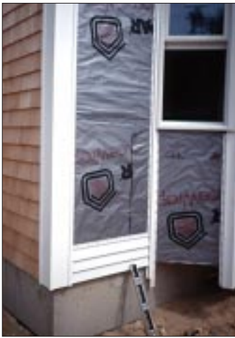
Figure 4. At a corner where cedar shingles and vinyl siding meet (left), the author uses \frac{7}{8} -inch J-channel to support the vinyl corner boards. On the vinyl-sided wall, he adds a second \frac{5}{8} -inch J-channel (right) to compensate for the vinyl's narrower profile.
