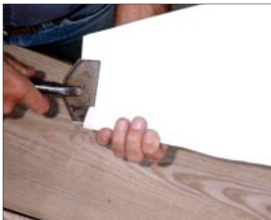
Figure 1. The author uses inexpensive, rough-cut fence boards to back the vinyl corner posts and aluminum rake and fascia. Aluminum trim pieces are attached with nails; the seams are sealed with silicone caulk and fastened with rivets.
