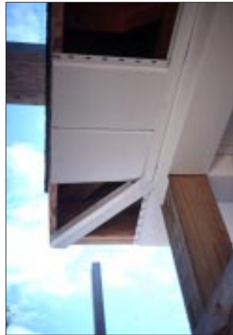
Figure 5. When installing aluminum soffit, the author leaves \frac{3}{8} inch for expansion inside the F-channel.
