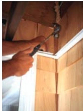
Figure 3. F-channel is an accessory that supports the aluminum or vinyl soffit where it meets the house. On shingled walls (above), the F-channel goes on after the shingles, flange up. With vinyl siding (left), the F-channel goes up first, flange down, and can support an optional crown molding.
