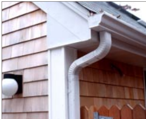
Figure 6. The aluminum rake returns (left) lap over the ends of the soffit and bend around the end grain of the wood rake and the back of the wood return. The aluminum rake and fascia then lap over the aluminum return (right).
