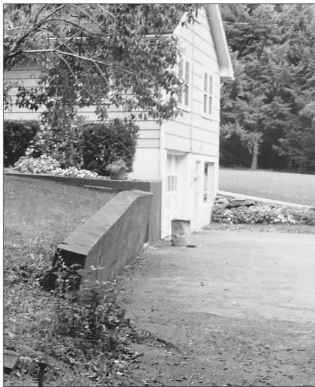
Figure 3. In northern climates, the freeze-thaw cycle is the primary cause of retaining wall failure. Wet soil expands as it freezes, exerting enormous force against the wall, pushing it outward. As the soil thaws, it settles into the space against the wall and the cycle is set to begin again with the next frost. With poured concrete walls, the entire wall often tips as a whole (left). In the case of block walls (center) or mortared stone walls (right), cracks and bulges may appear as sections of the wall tip.
