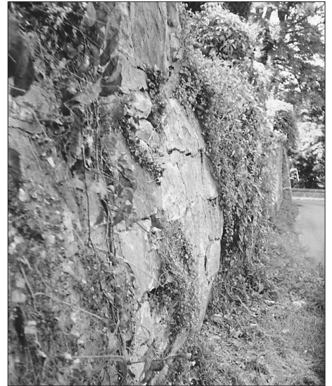
Figure 3. In northern climates, the freeze-thaw cycle is the primary cause of retaining wall failure. Wet soil expands as it freezes, exerting enormous force against the wall, pushing it outward. As the soil thaws, it settles into the space against the wall and the cycle is set to begin again with the next frost. With poured concrete walls, the entire wall often tips as a whole (left). In the case of block walls (center) or mortared stone walls (right), cracks and bulges may appear as sections of the wall tip.
