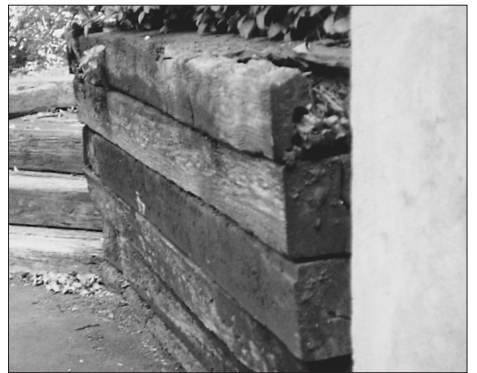
Figure 6. Railroad ties stacked and spiked together, but without tiebacks into the earth behind, cannot resist the force exerted by wet or frozen soil. Poor drainage also accelerates rotting.
