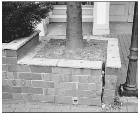
Figure 5. Tree roots can cause retaining walls to lean; keep large or fast-growing trees away.
