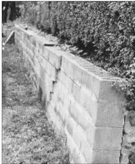
Figure 3. In northern climates, the freeze-thaw cycle is the primary cause of retaining wall failure. Wet soil expands as it freezes, exerting enormous force against the wall, pushing it outward. As the soil thaws, it settles into the space against the wall and the cycle is set to begin again with the next frost. With poured concrete walls, the entire wall often tips as a whole (left). In the case of block walls (center) or mortared stone walls (right), cracks and bulges may appear as sections of the wall tip.
