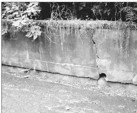
Figure 4. Shear failure occurs when the force of the soil causes the retaining wall to slide along a mortar joint, but without tipping over.
