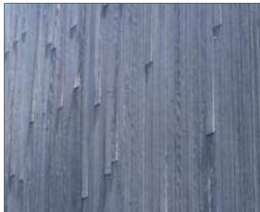
Figure 3. Use horizontal blocking at the joints in vertical siding. Otherwise, the end joints will pull loose and flap in the breeze — even with T&G, as shown here.
