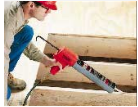
Figure B. Pneumatic guns, like the Rigid Power-Push, come in 10-ounce and 1-quart models and can be used with any compressor. Pressure is applied to the tube when you squeeze the trigger.
