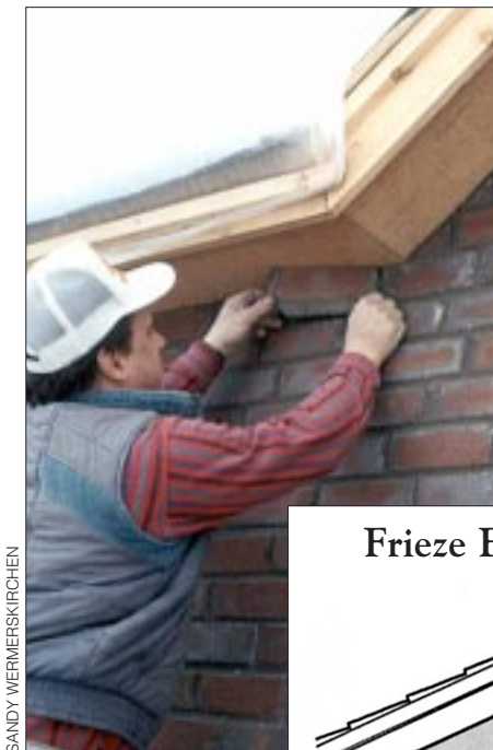
Figure 4. The author uses an oversize ruler, marked with letters rather than numbers, to gain or lose height incrementally. The higher the letter used, the greater the height of each course. By adjusting course height, the author minimizes cutting of bricks below window sills and soffits or above headers.
