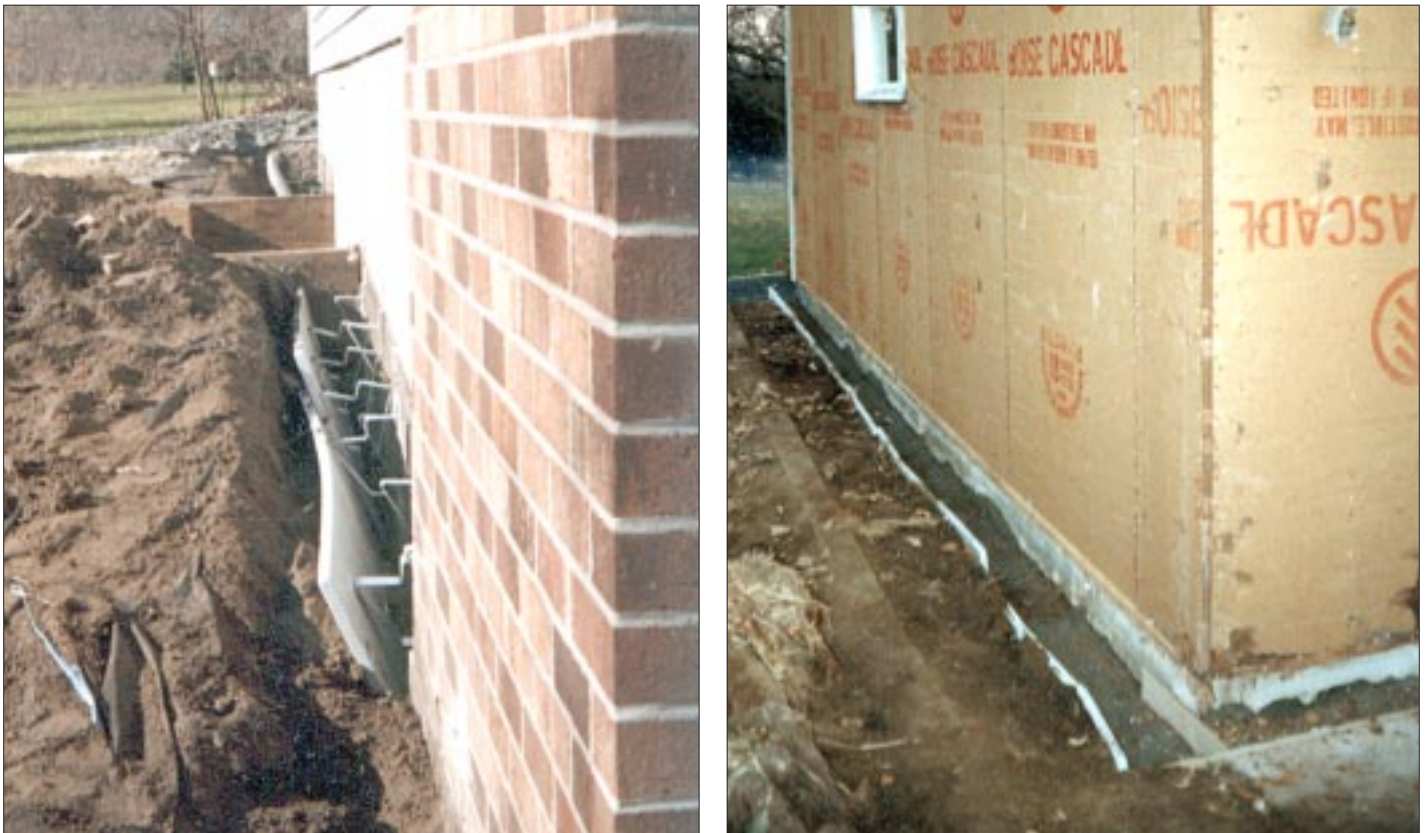
Figure 2. For retrofitting brick veneer, the author likes the Haunchomaster system, which creates a reinforced concrete shelf on an existing block foundation at grade level. Steel brackets are inserted into holes punched in the block, and joined horizontally with double rebar (left). Extruded polystyrene forms are attached to the angled face of the brackets. The finished shelf (right) can support a brick wall 18 feet high.
