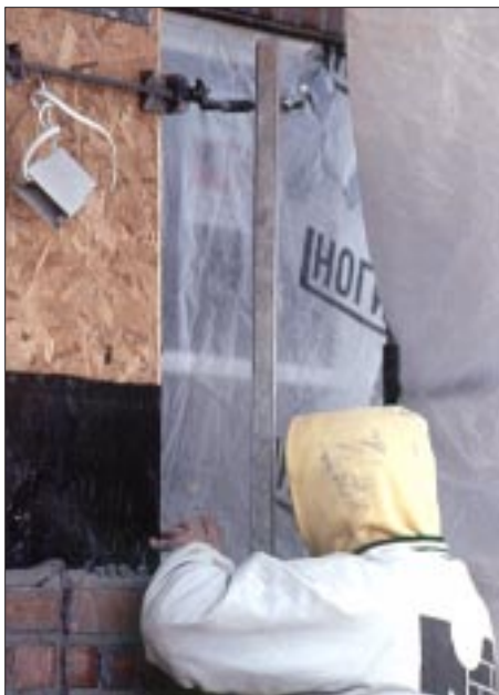
Figure 3. The author speeds production of decorative quoins by using a bracket-mounted aluminum jig called a Speed Lead (left). Bricks that make up the corners of the quoin are tucked into the corner of the device, establishing a plumb corner and a perfect reveal (right). The lead can be marked with a pencil to establish the height of each course of brick.
