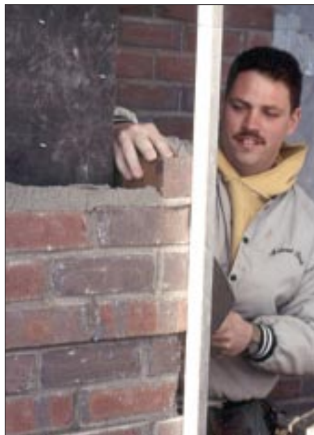
Figure 3. The author speeds production of decorative quoins by using a bracket-mounted aluminum jig called a Speed Lead (left). Bricks that make up the corners of the quoin are tucked into the corner of the device, establishing a plumb corner and a perfect reveal (right). The lead can be marked with a pencil to establish the height of each course of brick.
