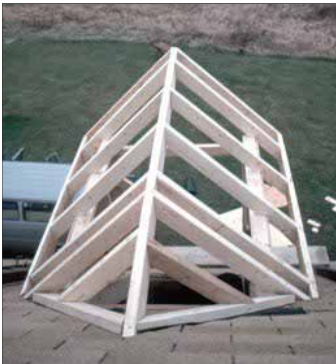
Figure 4. Use a plate to catch the edge of the roof sheathing in the valley, and to provide solid nailing for jack rafters (left). Where the dormer eaves intersect the main roof, provide a rafter with a bevel cut that matches the main roof pitch (above).
