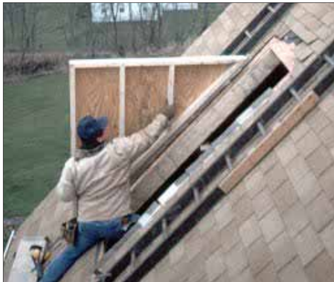
Figure 2. To reduce the amount of time the attic is exposed to the weather, frame the dormer opening from the inside and prebuild the walls. After cutting away the sheathing, pass the prebuilt walls through the opening (left), and install them in one piece (right).
