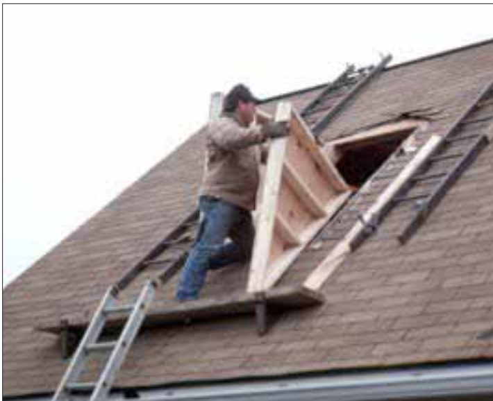
Figure 2. To reduce the amount of time the attic is exposed to the weather, frame the dormer opening from the inside and prebuild the walls. After cutting away the sheathing, pass the prebuilt walls through the opening (left), and install them in one piece (right).
