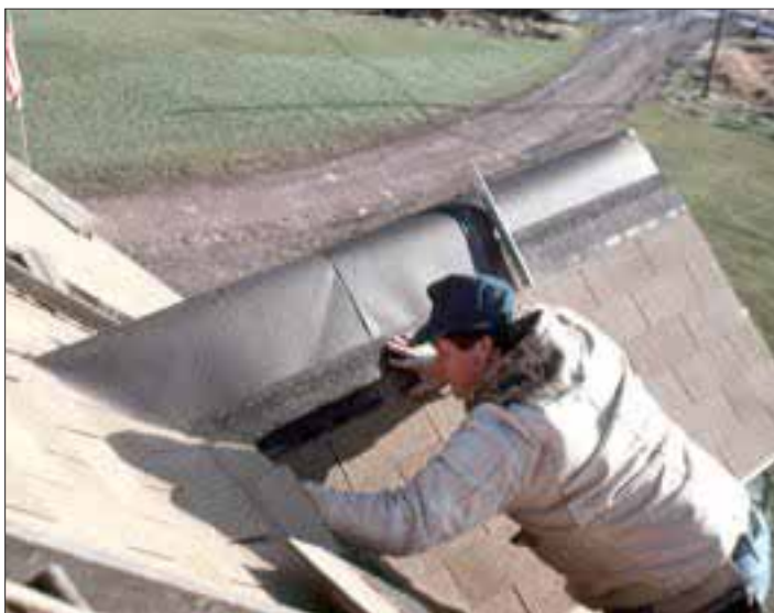
Figure 5. When roofing the dormer, slide the new shingles up under the existing ones. This eliminates the need for a perfect cut on the dormer shingles and gives extra protection at the new valleys.
