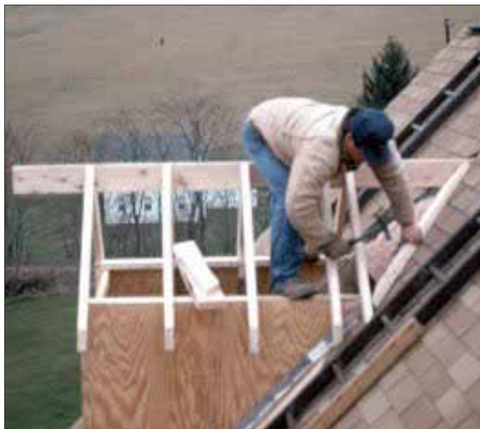
Figure 4. Use a plate to catch the edge of the roof sheathing in the valley, and to provide solid nailing for jack rafters (left). Where the dormer eaves intersect the main roof, provide a rafter with a bevel cut that matches the main roof pitch (above).
