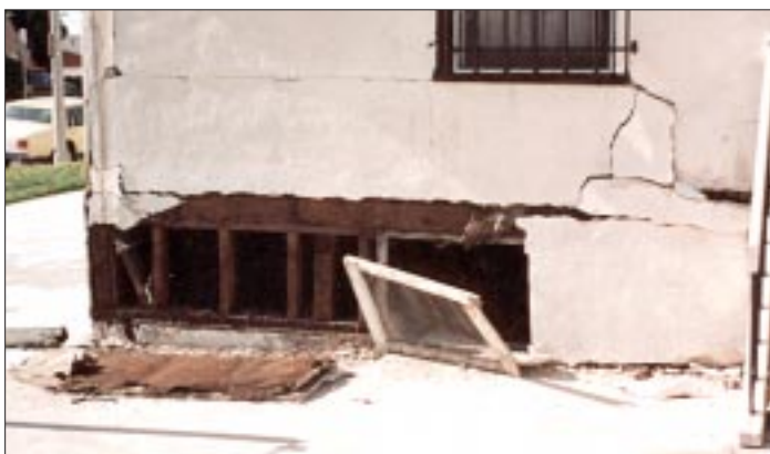
Although this stucco damage looks severe, this house is still structurally sound.
