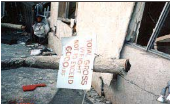
Bent-over columns and severed connections bear witness to the earthquake's powerful jolting shocks. The steel column shown here contained no concrete.
