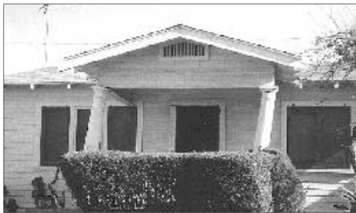
Leaning porch posts are a sign that this house has jumped off its cripple walls.
