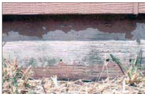
Masonite says faulty installation and maintenance caused problems with its product in South Florida. The siding shown here was installed in contact with the ground.
