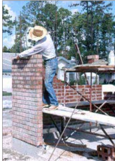
SuprKing structural bricks are slightly oversize and have large holes for grout and rebar. Here a mason works on a reinforced load-bearing brick wall.
