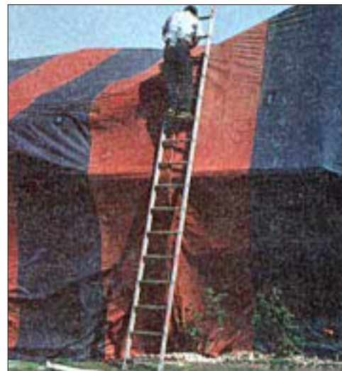
Fumigation techniques that require the whole house to be covered with a tarp proved most effective in head-to-head termite control tests.
