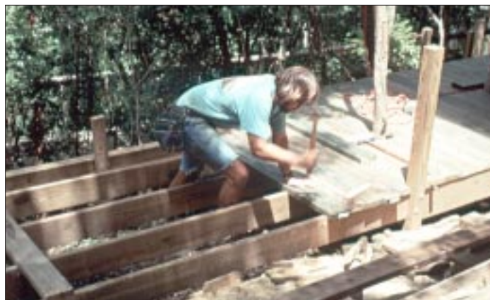
ACQ Preserve, the new pressure-treated lumber product that contains no arsenic or chromium, now carries a "green label" certifying its environmental advantages.
