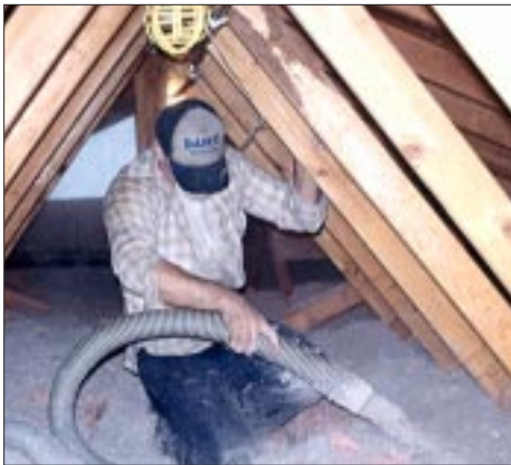
An added layer of blown-in cellulose will eliminate convective losses in attics insulated with loose-fill fiberglass, researchers say.
