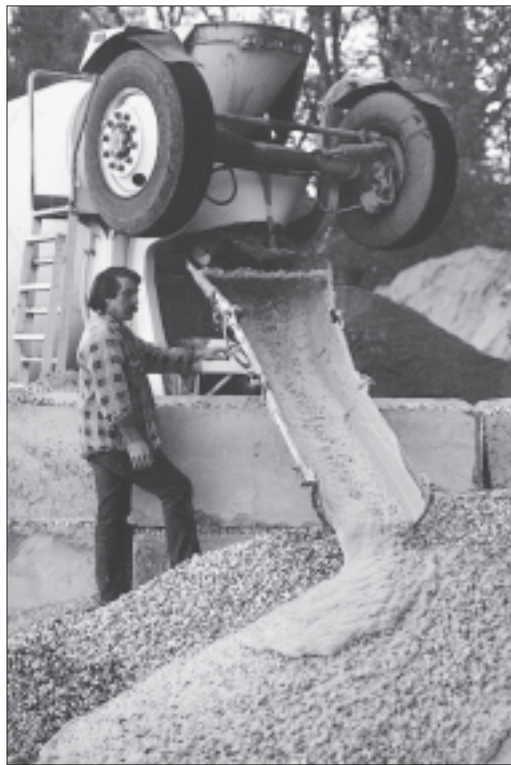
Contractors in Colfax, Calif., mix gravel or sand with water and soap to create a sudsy, flowable mix.
