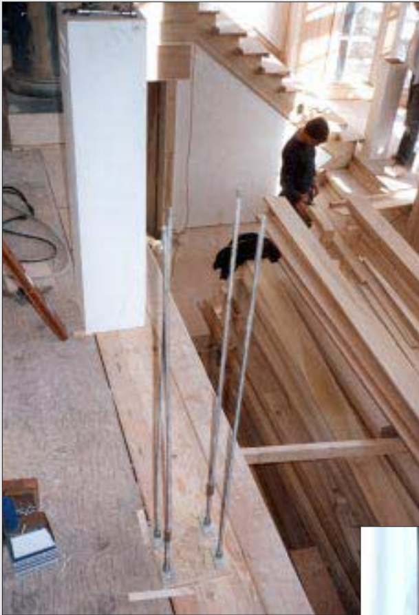
Figure 6. The author secured these hollow newels (right) to the floor with hardwood blocks, plumbing pipe hanger plates, and \frac{5}{16} -inch threaded rods (see detail, above right). In the photo above, the threaded rods have been fastened to the hanger plates and are waiting for the hollow newel to be slipped into place.
