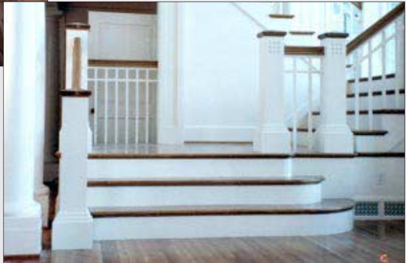
Figure 6. The author secured these hollow newels (right) to the floor with hardwood blocks, plumbing pipe hanger plates, and \frac{5}{16} -inch threaded rods (see detail, above right). In the photo above, the threaded rods have been fastened to the hanger plates and are waiting for the hollow newel to be slipped into place.
