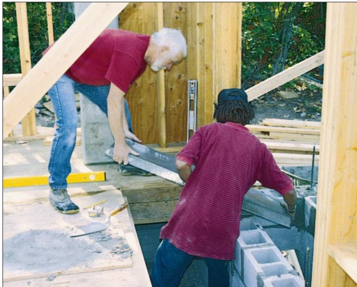
Figure 5. Common in the Northwest, corbel slabs are even quicker than block and steel hearths. Here, a pair of masons set the first hundred-pound corbel slab into place (left). Within an hour, the hearth base is complete (below).
