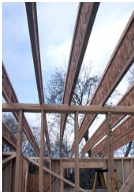
Figure 4. Wood I-joists tend to bow — if you aren't careful, you can push and pull an I-joist into an S-shape when nailing decking.
