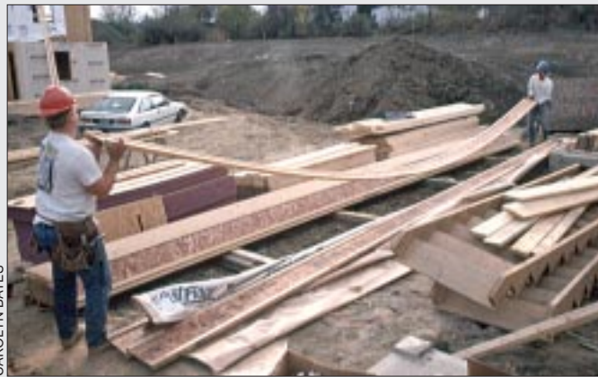
Figure B. Wood I-joists are light enough for one man to carry, but they're so flexible — especially long ones — that handling them is two-man work.
