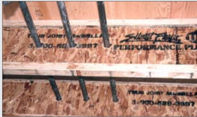
Figure A. The prepunched knockouts in wood I-joists don't always line up and often aren't where you need them. But the 1/2-inch web is easier to drill than sawn lumber.
