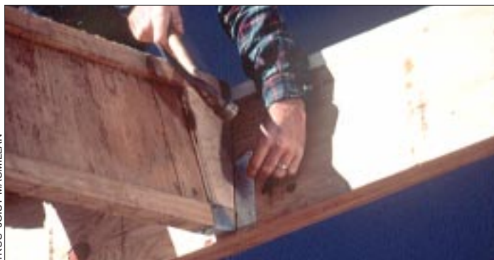
Figure 3. The web of the wood I-joist must be padded out when joist hangers don't support the top flange.
