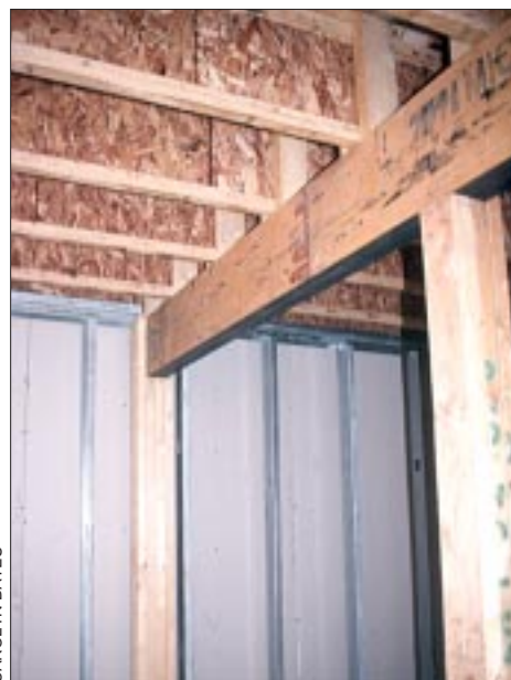
Figure 2. Wood I-joists need "squash blocks" to support point loads or bearing walls (left). Extensive blocking is also necessary at cantilevers and where bearing walls are offset (right).
