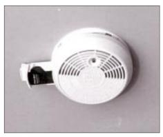
Carbon monoxide detectors resemble ordinary smoke detectors. They cost from \$40 to \$80 and are available in 110-volt, 12-volt, or battery-powered versions.
