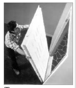
The Secura-Fit replacement door is similar in concept to a replacement window in that it gives you a new exterior door with minimal fuss. The product consists of an insulated 18-, 20-, 22-, or 24-gauge galvanized steel door hung in a 16-gauge adjustable steel jamb. It's insulated with a high-density polyurethane core, and made weathertight by a magnetic weatherstripping system and an adjustable door sweep.
