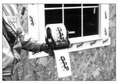
happens at sheathing joints and around door and window frames, housewrap makers want you to wrap the entire house. And some research has suggested that real energy savings comes only when you tape the seams on the housewrap.
