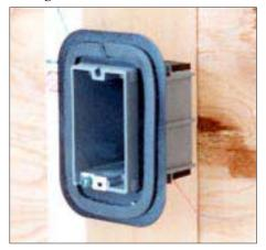
If you're an air-sealing nut, you probably worry about your electric outlets. Air escaping through exterior wall outlets can raise a home's heat loss and carry moisture into the wall cavity. In very cold climates, this moisture can condense inside the cavity, causing all sorts of mischief.
