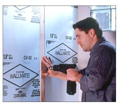
entire wall, the rabbets form a series of 2-foot on-center channels that are just big enough for 1x3 furring strips, which can then be fastened through the insulation and into the wall with Tapcontype screws. The furring strips hold the insulation in place and act as a screw base for drywall.
