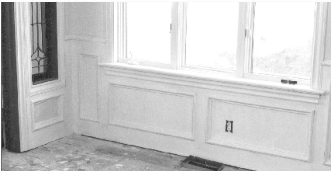
In a well-designed wainscot installation, the edges of the rectangular panels line up with the edges of the window casings, and the widths of the stiles and rails all match.
