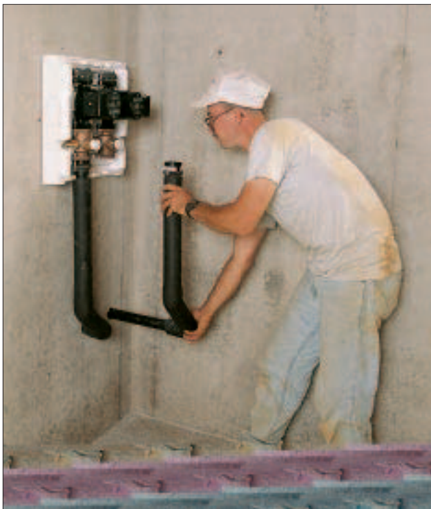
Figure 3. In the basement, the author's son connects the end of the ground loop to a manifold (above), then fills the loop with coolant and purges the air from the system (right).
