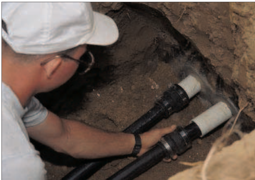
Figure 2. Plastic pipe for the ground loop penetrates the foundation wall below the frostline (above). A rubber clamp secures the pipe to the PVC sleeve in the foundation wall. All T-joints in the ground loop pipe are made with an electric heat-fusing tool — mechanical or glued joints will not hold up (left).
