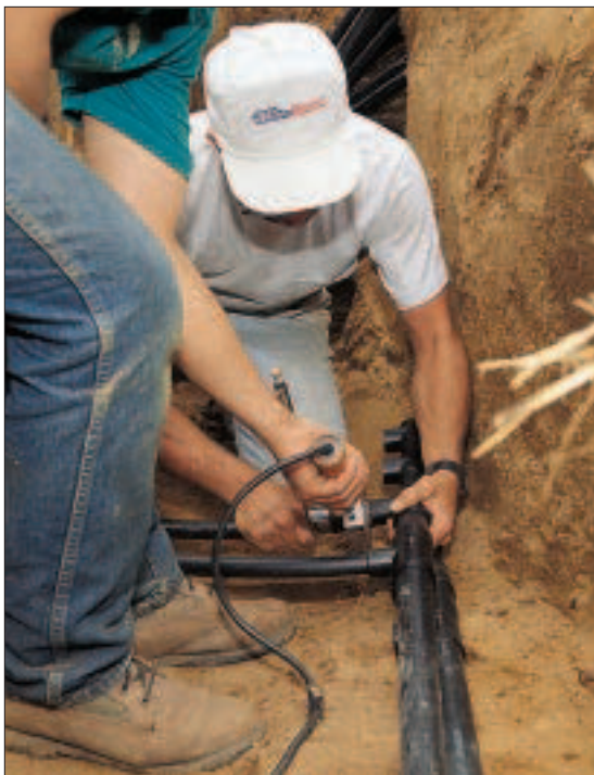
Figure 2. Plastic pipe for the ground loop penetrates the foundation wall below the frostline (above). A rubber clamp secures the pipe to the PVC sleeve in the foundation wall. All T-joints in the ground loop pipe are made with an electric heat-fusing tool — mechanical or glued joints will not hold up (left).
