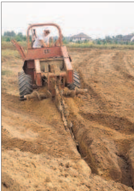
Figure 1. To put in a ground loop, the author digs several hundred feet of trench (left). On smaller lots, ground loops can be installed in vertical boreholes (right).
