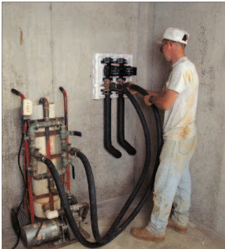
Figure 3. In the basement, the author's son connects the end of the ground loop to a manifold (above), then fills the loop with coolant and purges the air from the system (right).
