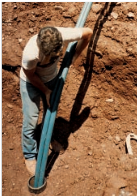
Figure 1. To put in a ground loop, the author digs several hundred feet of trench (left). On smaller lots, ground loops can be installed in vertical boreholes (right).
