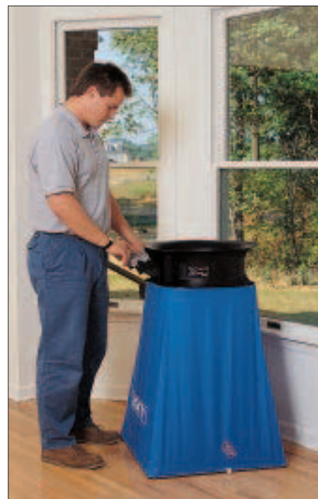
Figure 5. Utilities will only guarantee a rebate for a ground-source system if the ductwork passes a duct-blasting test.
