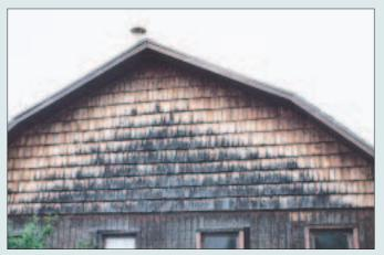
"Extractive bleeding" has streaked these shingles below the nail holes (top). Iron in nails can react with natural wood tannins to make bleeding worse. Bleeding stains can also emerge from wood grain, even on stained or painted siding (middle). Bleeding is caused by water — note that the shingles protected by the eaves show less staining (bottom).
