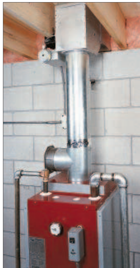
Figure 3. Combustion-air kits, such as the In-Forcer by Tjernlund, usually use a 50-cfm fan to bring outside air directly to the burner. Special controls turn the air-supply fan on whenever the burner fires.
