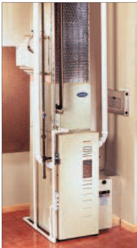
Figure 1. Like many high-efficiency condensing furnaces, Carrier's WeatherMaker uses plastic pipe both to vent through the sidewall and to bring combustion air to the burner. The acidic condensate is also carried away in plastic drain piping.
