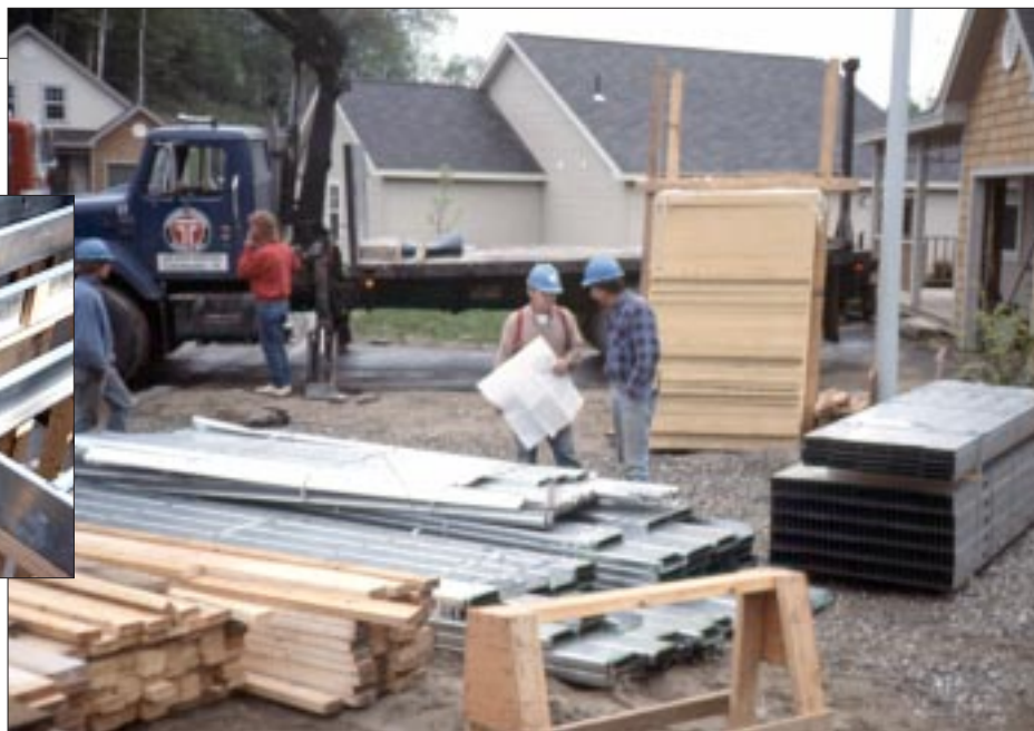
Bundles of wood studs and steel joists await use in a hybrid frame.
