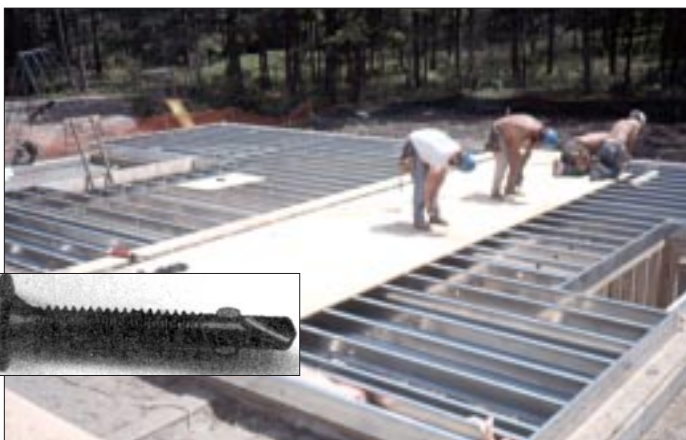
Figure 5. The author's crews use special self-tapping screws for attaching plywood subflooring to steel joists. The wings on the screw tip clear the plywood shavings so the threads don't clog, then shear off when they hit the joist.
