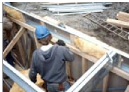
Figure 3. Because steel is much more heat-conducting than wood, the author uses wood studs for exterior walls. The steel band joist is backed with a ripped 2x10, and stuffed with batt insulation for an extra measure of thermal protection (inset).
