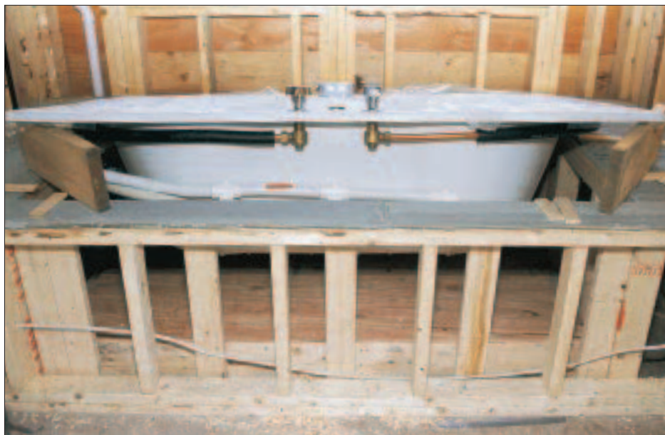
Figure 4. After lifting the tub into place to test the fit, the author lifts it out again to lay wet mortar under the base.
