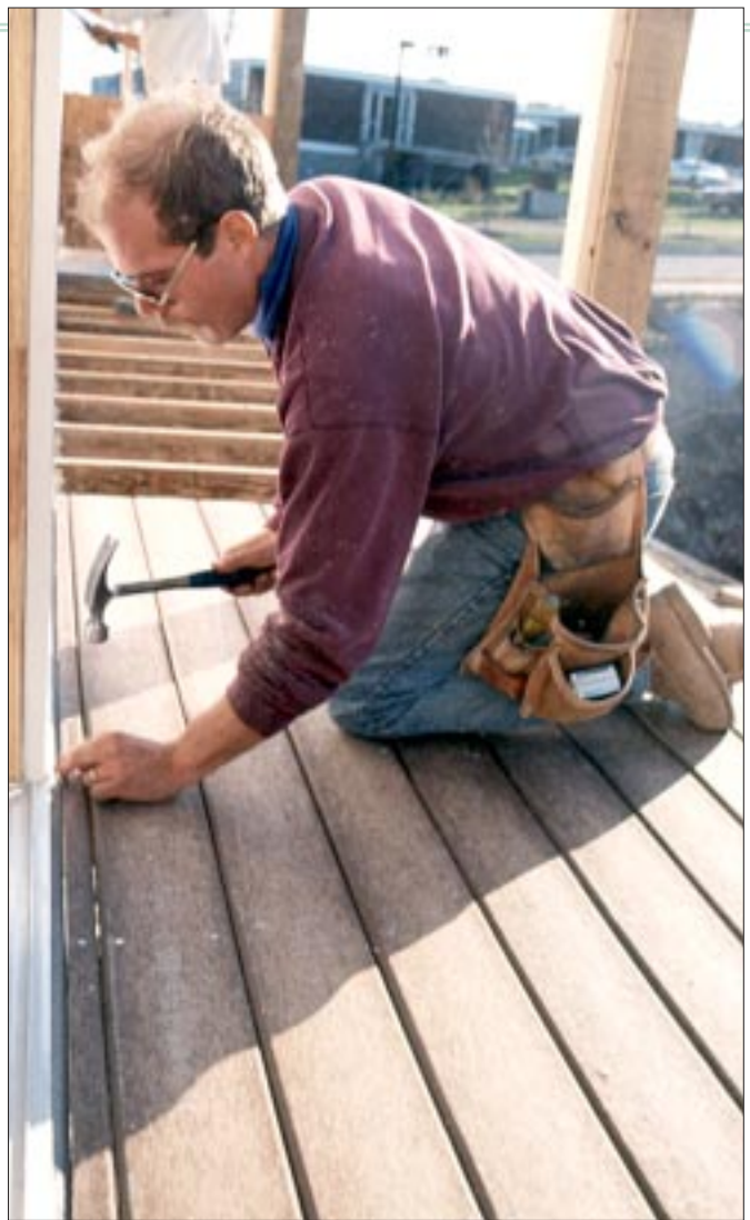
Trex provides a splinter-free alternative to wood decking. The wood-plastic composite can be nailed close to its edge without splitting.
