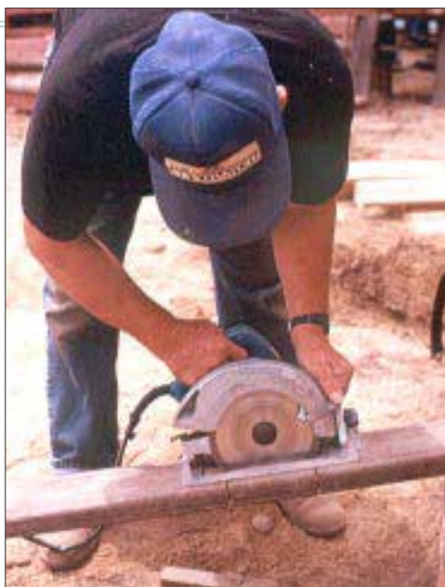
Trex cuts as easily as wood with a circular saw. It can also be drilled, sanded, and powerplaned like wood.
