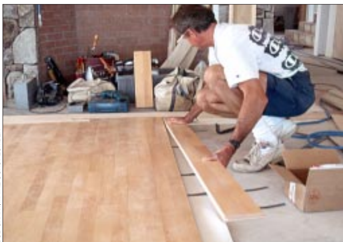
Figure 2. The Junckers floating floor system uses metal clips to hold the thick hardwood strips together. You can remove the floor by unsnapping the clips.
