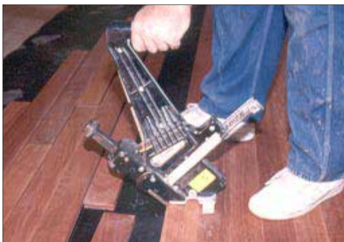
Figure 3. To prevent the nails from striking the concrete, the author places shims under the foot of the nailing machine when he has to nail into a 1/2-inch plywood subfloor.
