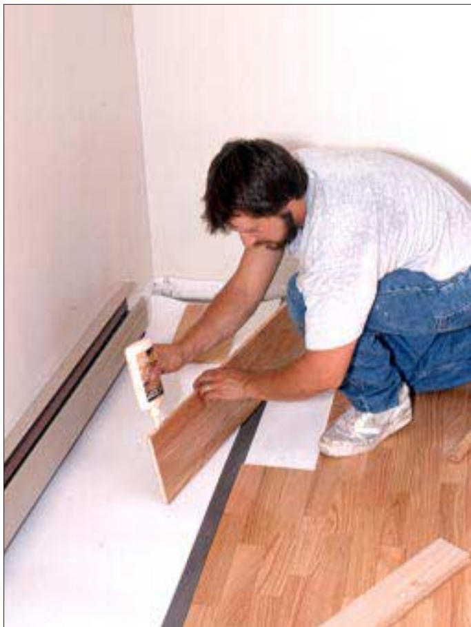
Figure 1. Floating laminated plank floor sections are edge-glued to each other and laid over a foam pad. The floor is said to "float" because it isn't fastened to the subfloor — only gravity holds it down.
