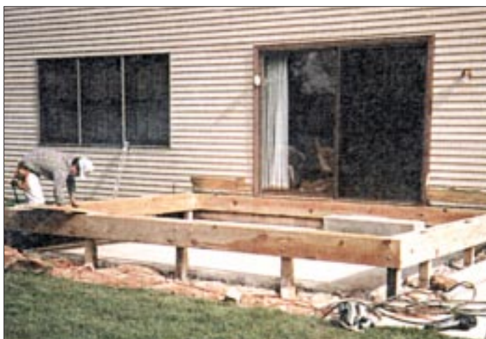
Figure 4. Here, posts 4 feet on-center and a double rim joist are added around an existing concrete patio (left). The author removed only as much concrete as necessary to dig the postholes. With the PT plywood skirt in place (right), the framed deck is ready to build on.
