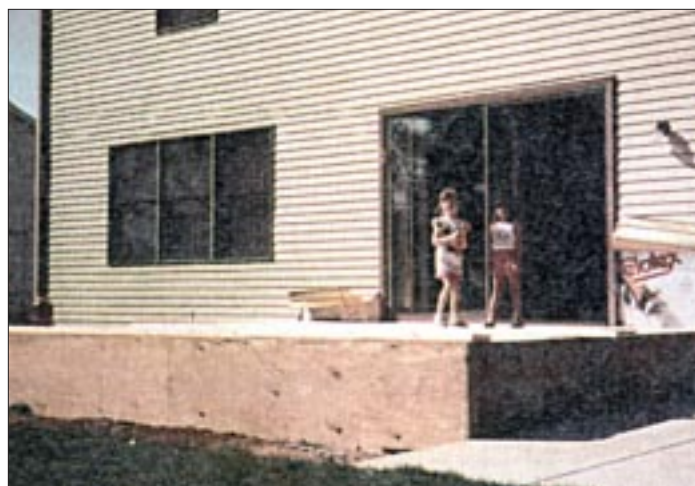
Figure 4. Here, posts 4 feet on-center and a double rim joist are added around an existing concrete patio (left). The author removed only as much concrete as necessary to dig the postholes. With the PT plywood skirt in place (right), the framed deck is ready to build on.
