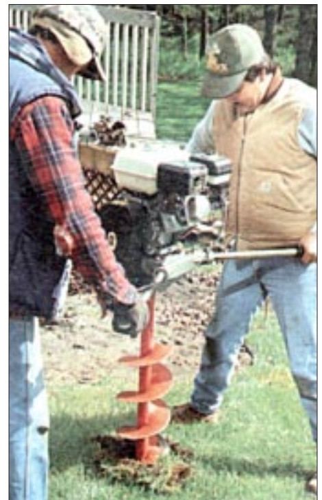
Figure 3. A two-man power auger speeds the digging of pier holes.
