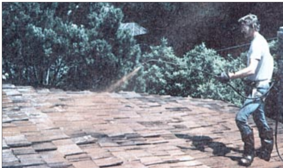
Figure 2. Untreated wood roofs can be protected by direct surface spraying of an approved fire-retardant chemical. Protection is temporary, however, since the fire retardant does not penetrate well into the wood surface, and the active chemical leaches quickly in the rain. Some formulas dissipate completely within a few months.
