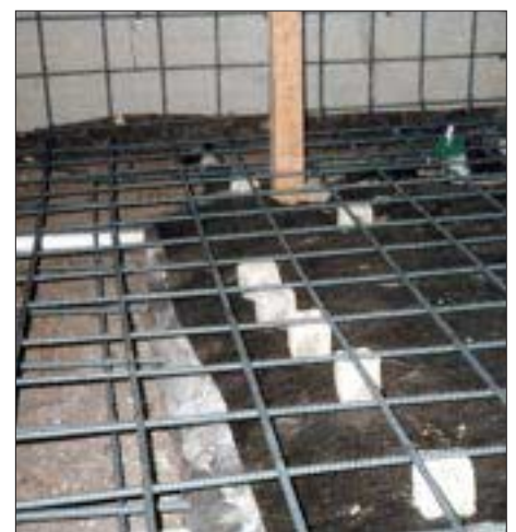
Figure 3. Concrete “dobies” are used to hold rebar off the ground or away from forms, ensuring adequate concrete coverage and preventing rust.
