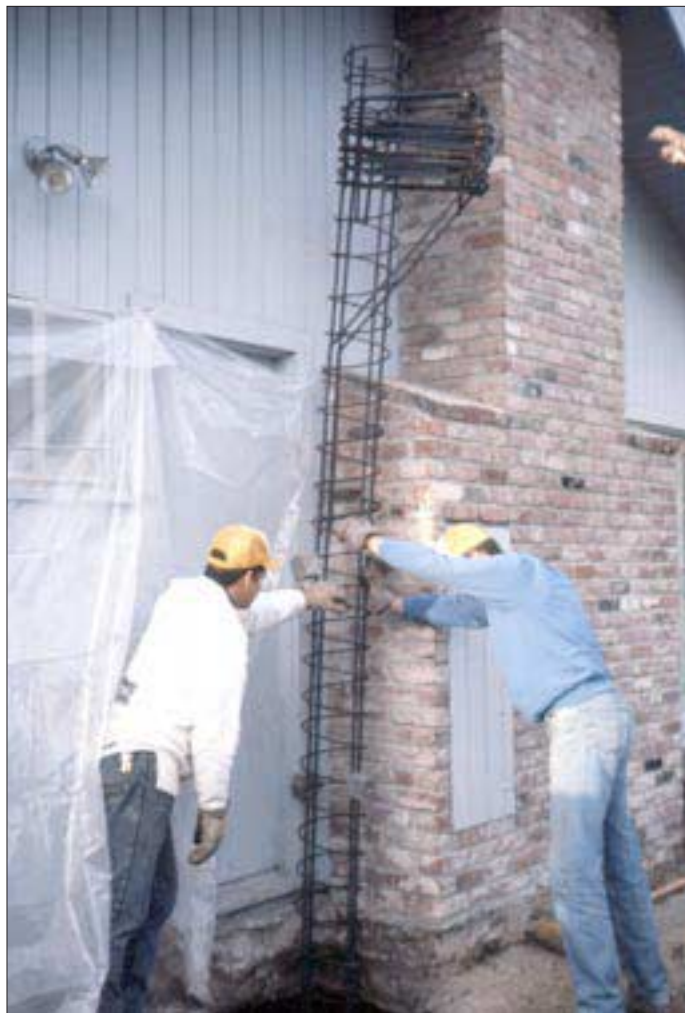
Figure 1. For deep concrete piers, the author uses steel cages made from #3 rebar spirals with #5 rebar in the middle. The cage shown here will help support the brick chimney in a foundation underpinning job.
