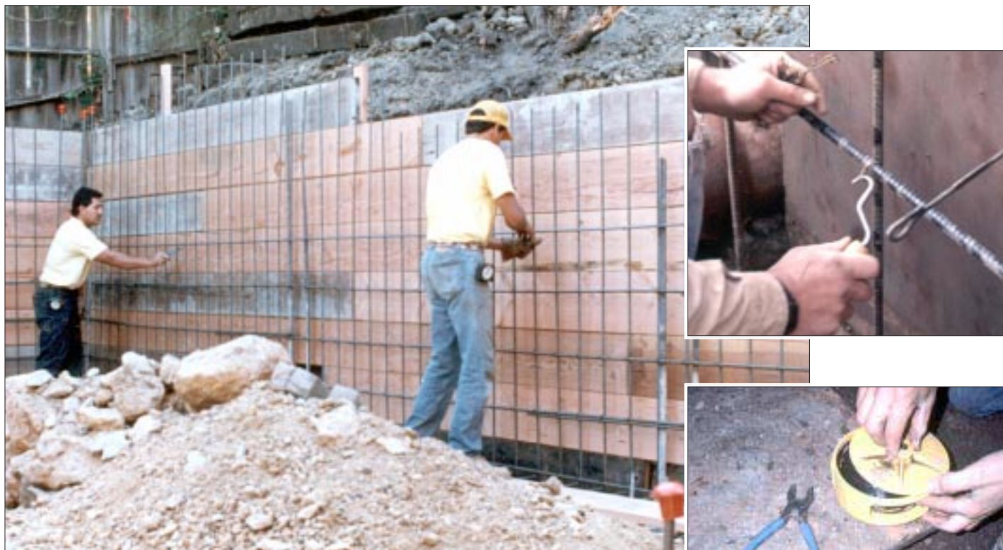
Figure 4. The author ties the rebar at every intersection. Precut wire can be bought in bundles and twisted with a special swiveling tool (top right), but the author's crew prefers to use a pair of spring-loaded linesman's pliers and a roll of wire on a spool (right).
