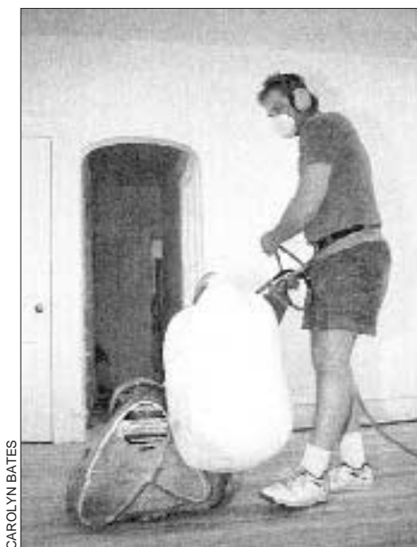
To blend patched hardwood flooring, you may need to sand and refinish the whole room.
