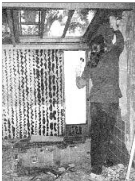
Removing mortar-base tile takes more time than stripping tile from drywall.
