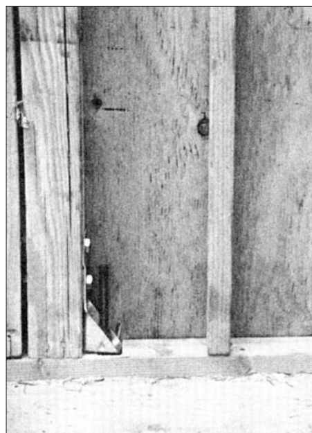
Figure on extra labor to bolt shear walls to the foundation.
