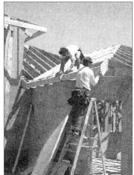
Roofs with hips and valleys are more expensive to frame and finish than gable roofs.
