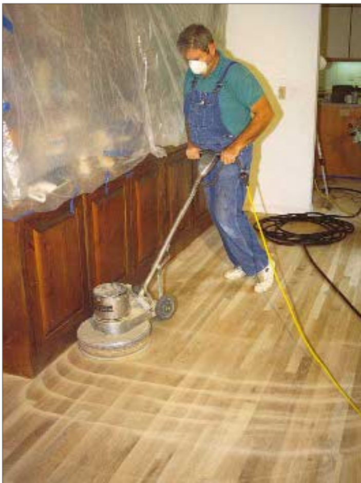
Figure 5. A last run with a buffer/polisher removes the overlap between the areas you did with the drum sander and edger. Screening will not remove drum marks or deep scratches from the edger, however — they'll reappear as soon as you apply the finish.
