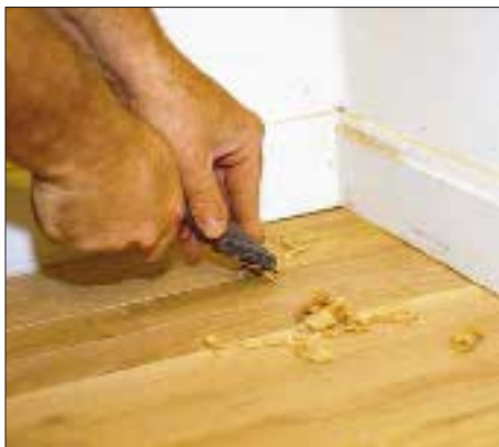
Figure 4. Remove finish from out-of-the-way corners by holding a scraper flat against the floor, and pulling with firm pressure. Be careful not to allow the corners to dig in, and always work with the grain.
