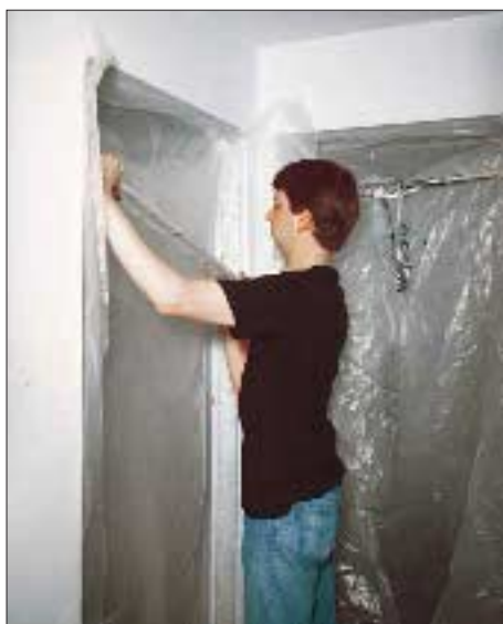
Figure 2. To seal halls or doorways, the author builds friction-fit frames from strapping and poly. Vertical pieces cut just short of doorway height are held in place by horizontal pieces cut \frac{1}{8} -inch long. The frames can be assembled or disassembled in less than a minute.
