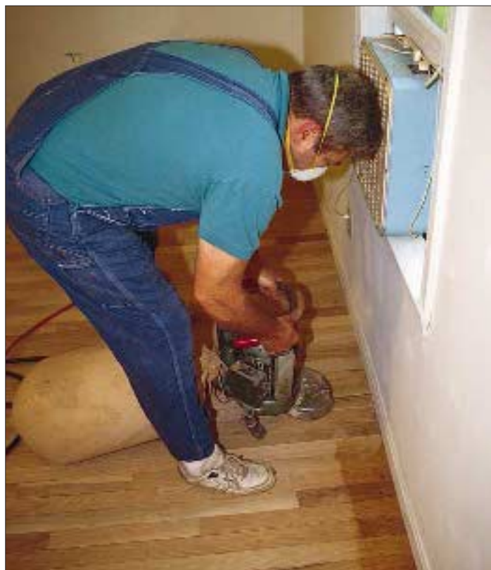
Figure 3. The circular motion of the edger cuts across the grain, and digs into the wood more easily than a drum sander. To avoid damage, move the edger in an elliptical motion with the long axis parallel to the grain.
