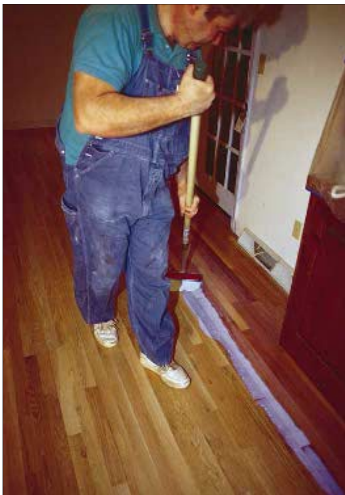
Figure 6. To apply the finish, the author uses a foam paint applicator on a long handle. He holds the mop at a slight angle to both work the finish into the grain and keep the excess out in front on the bare floor.
