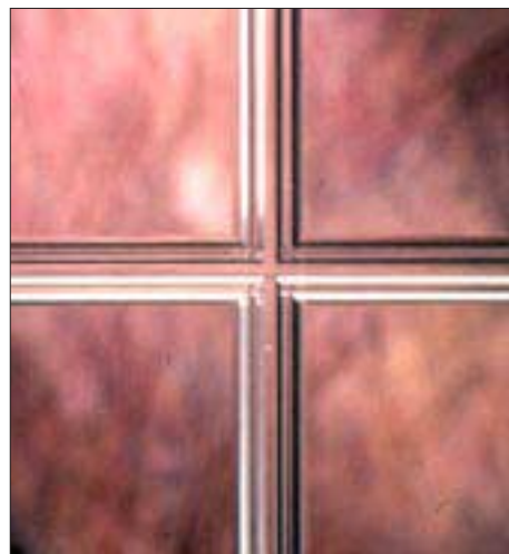
Figure 4. Instead of true divided lights or clip-on grilles, Eagle's Decorelle 150 glazing has a clear or frosted groove cut into its face.
