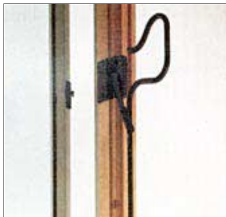
Figure 2. For those who have trouble opening casement locks, Andersen's optional tandem sash lock (left) makes it easy to operate both locks at the same time. Andersen's custodial sash lock (right) can prevent small children from opening a casement. It can only be unlocked with an allen wrench or a tool supplied by the company.
