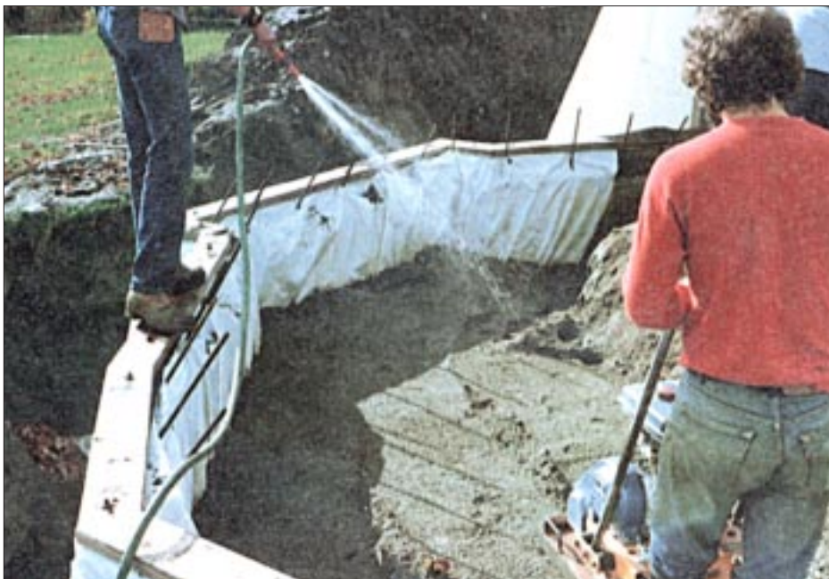
Figure 2. The large surface area of a vibratory plate compactor works well with sand and gravel. Here a worker moistens dry sand to speed compaction. The small footprint of a jumping jack (right) does a good job of compacting, particularly in tight spaces. Note the red horizontal lines on the foundation wall, used to estimate the thickness of each lift of soil.
