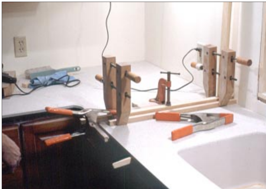
Figure 4. The countertop joint is clamped together using strips of hardwood attached to the two pieces with hot-melt glue. A clamp screwed to a plywood block, also fastened with hot-melt glue, holds the two surfaces flush.
