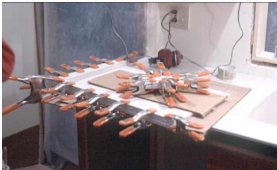
Figure 5. Counter edges are built up with two 1/2-inch strips of Surell, seamed together with compound and thoroughly clamped to minimize joint lines (above). Trimming with a router and straightedge yields a smooth, one-piece finish (left).
