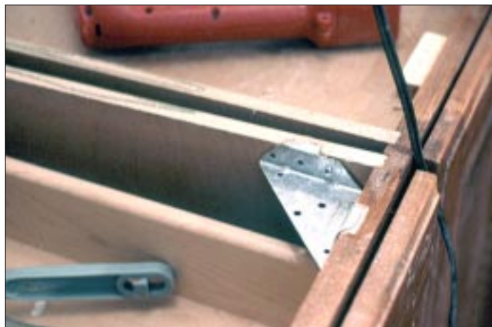
Figure 1. Modifying the stock cabinets. Solid surface counters must be well supported from underneath. To match the one-inch buildup on the front edge of the counter, the author added a continuous one-inch-thick wood strip to the top of the cabinets along the wall and crosswise at every cabinet side (left). To provide a perfectly smooth bearing, he also had to recess the cabinets' metal corner brackets (right), which protruded above the top surface of the cabinets.
