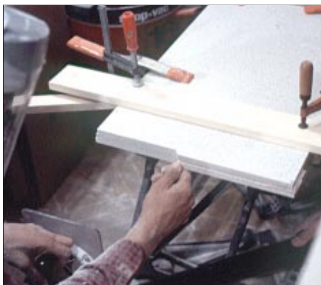
Figure 5. Counter edges are built up with two 1/2-inch strips of Surell, seamed together with compound and thoroughly clamped to minimize joint lines (above). Trimming with a router and straightedge yields a smooth, one-piece finish (left).
