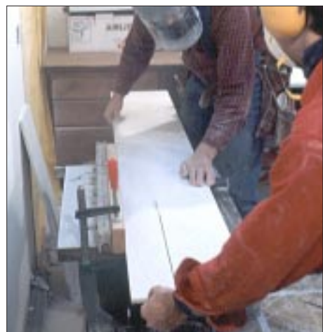
Figure 2. Solid surfacing can be cut with standard woodworking tools equipped with carbide-tipped blades. Here, the author rips a piece of Surell on a portable table saw.
