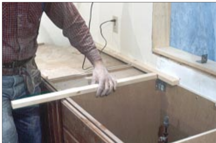
Figure 1. Modifying the stock cabinets. Solid surface counters must be well supported from underneath. To match the one-inch buildup on the front edge of the counter, the author added a continuous one-inch-thick wood strip to the top of the cabinets along the wall and crosswise at every cabinet side (left). To provide a perfectly smooth bearing, he also had to recess the cabinets' metal corner brackets (right), which protruded above the top surface of the cabinets.
