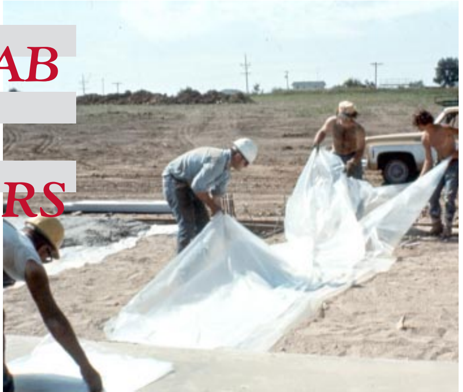
Workers place a vapor barrier over compacted sand before pouring a slab.
