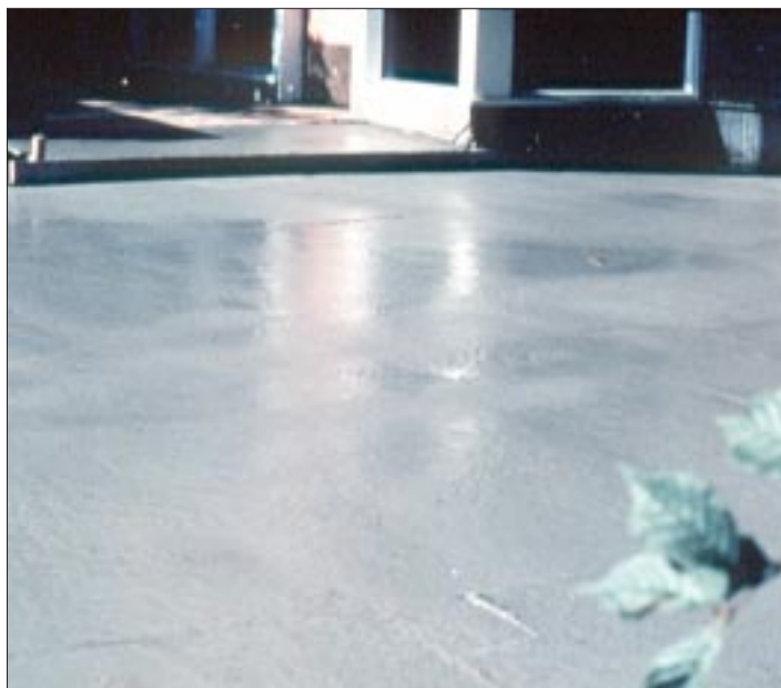
Figure 1. Placing a slab directly on a vapor barrier can cause excess bleed water to rise to the surface (top). Troweling the slab before all the bleed water has disappeared can cause surface defects, such as crazing (middle) and scaling (bottom).
