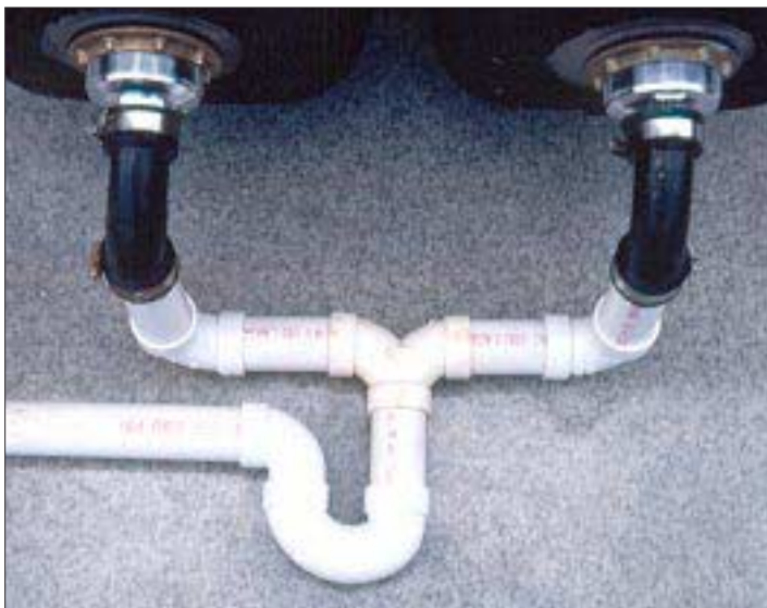
Figure C. For a leakproof drain and trap assembly, the author uses glued plastic fittings and places the pipes at the back of the sink cabinet. The rubber 90-degree elbows, attached with hose clamps, allow for quick disassembly.
