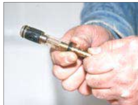
Figure L. This Delta single-lever faucet repair kit includes new springs and gaskets (left); for other faucet designs, such as the Moen, the entire cartridge is replaced (right).
