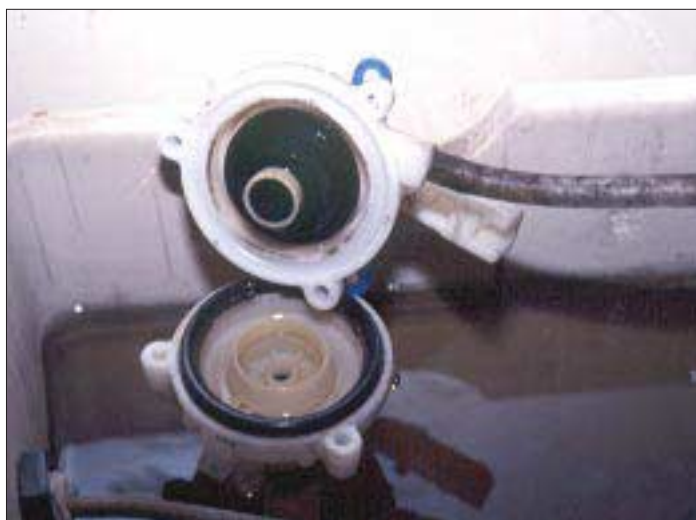
Figure G. Sometimes replacing the seal in the refill valve can remedy a running toilet. More often, though, the entire assembly must be replaced.
