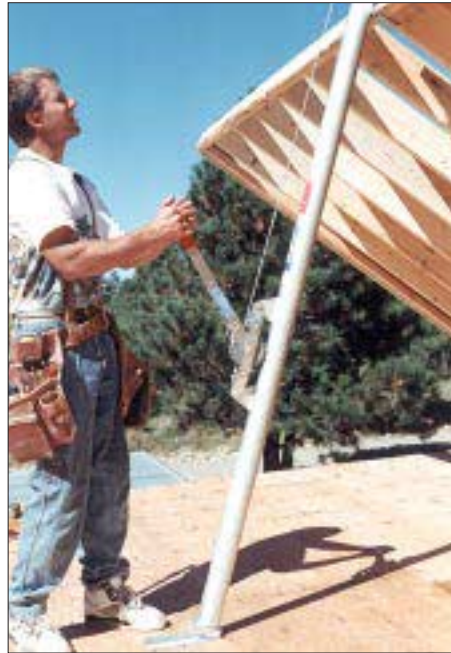
To lift framed walls safely and efficiently, a carpenter uses Proctor Wall Jacks.
