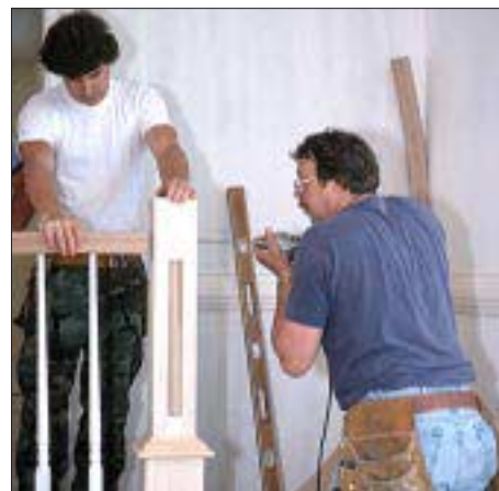
C. Blodgett predrills a hole for lagging the end of the curved railing to the newel post.
