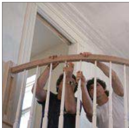
B. Many hands make tight work, as the predrilled railing slips into place.
