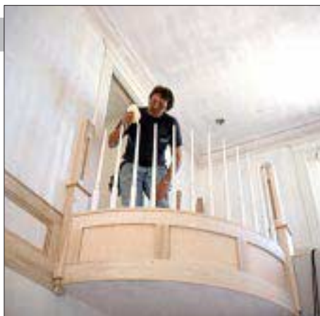
A. Bob Blodgett puts glue on the tops of the candlestick balusters in preparation for railing installation.
