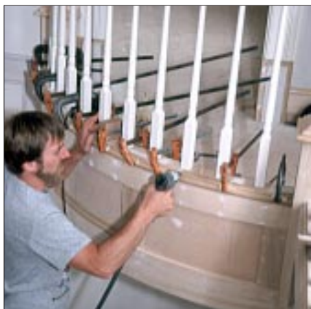
G. After coming off the form, the longer moldings are glued, clamped, and tacked in place.
