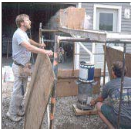
D. A kerosene heater with a metal can full of water on top supplies steam to the site-built 2x10 steam box.
