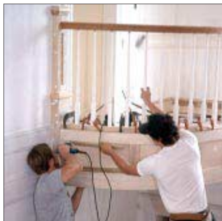
H. Because of their tendency to spring back, the shorter moldings must be attached with countersunk screws.
