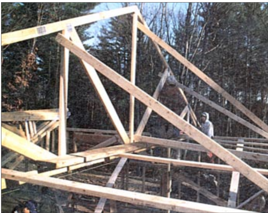
By starting truss installation several feet in from one end of the building and bracing back to the end wall, the author avoids using long bracing from the roof to the ground.
