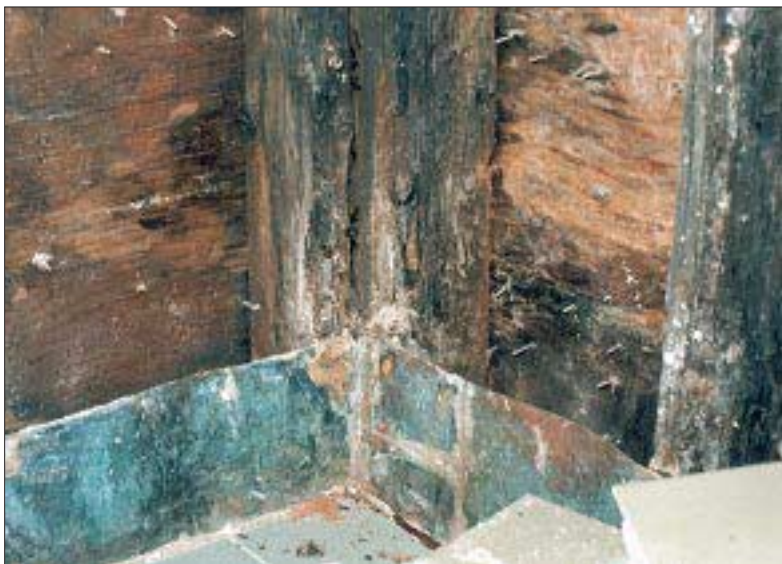
Figure 1. The framing behind this shower stall (above) rotted because bathroom moisture leaked into the walls. The excess moisture also caused extractive staining on the home's siding (right). The solution was to add a bath fan that vented moisture directly to the outside.
