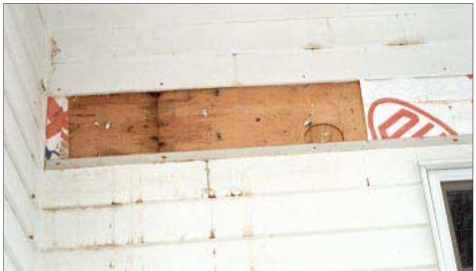
Figure 2. Water vapor from inside this new house — caused in part by green framing lumber and a dryer vented directly into the basement — leaked through the walls and caused extractive staining on the primed and painted siding (below).
