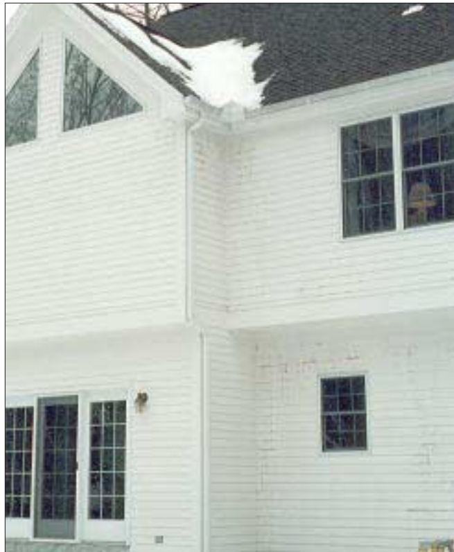
Figure 2. Water vapor from inside this new house — caused in part by green framing lumber and a dryer vented directly into the basement — leaked through the walls and caused extractive staining on the primed and painted siding (below).
