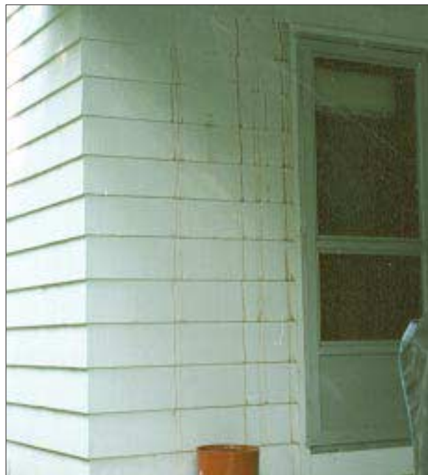
Figure 1. The framing behind this shower stall (above) rotted because bathroom moisture leaked into the walls. The excess moisture also caused extractive staining on the home's siding (right). The solution was to add a bath fan that vented moisture directly to the outside.
