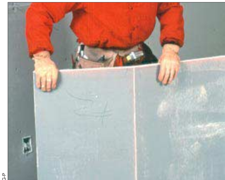
Figure 6. Scoring and snapping Dens-Shield leaves a very crisp edge. The material is also less brittle than cement-based backerboards, so it won't crack or crumble, even when cut into narrow strips.
