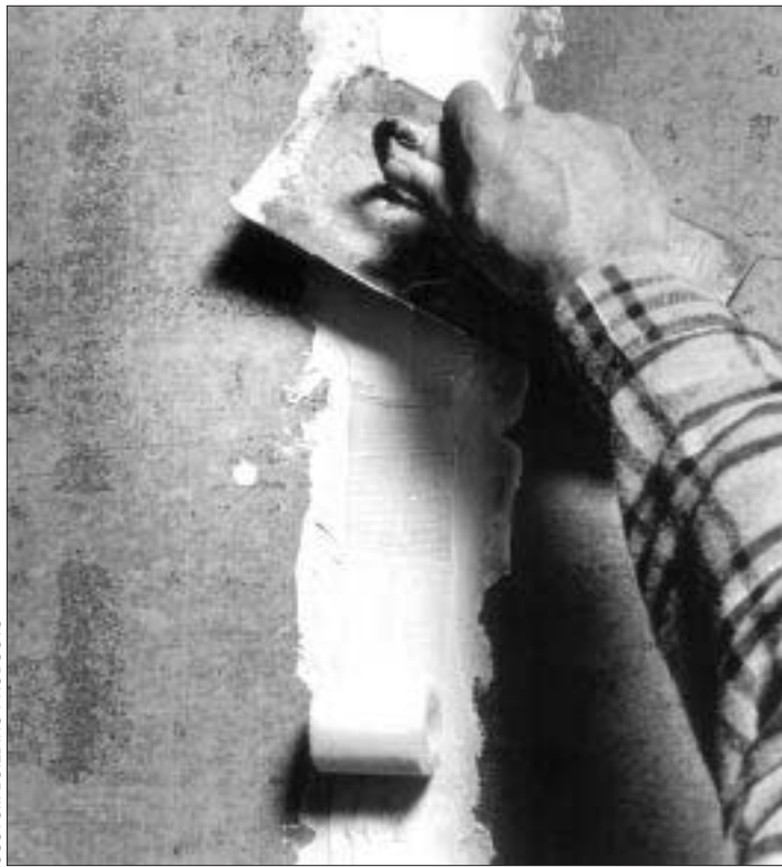
Figure 5. Seams in cementitious backerboard should be taped with fiberglass mesh bedded in dry-set or latex-modified Portland cement mortar.
