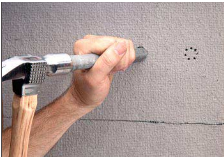
Figure 2. Cut small openings for pipes by using a masonry bit to drill a series of small holes at the perimeter, then punch through with a piece of pipe.
