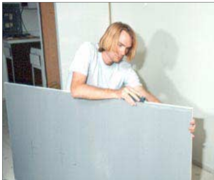
Figure 6. Scoring and snapping Dens-Shield leaves a very crisp edge. The material is also less brittle than cement-based backerboards, so it won't crack or crumble, even when cut into narrow strips.
