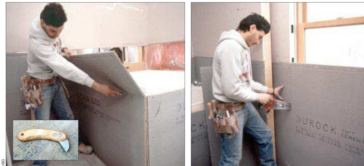
Figure 1. Backerboard can be scored and snapped like drywall (left). A carbide-tipped scoring tool (inset, left) will last longer, but the author prefers to use a utility knife because the cut is cleaner and more accurate. At door and window openings, a handsaw makes clean cuts (right). The saw teeth will dull quickly, however, so use a keyhole saw with replaceable blades.
