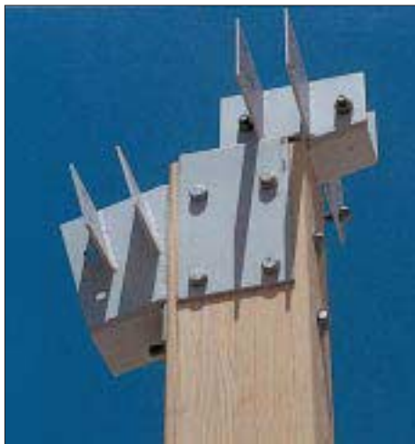
Figure 5. In metal side plate connections, such as the ones at the top of this glulam post (left), the bolts must be adequately sized to transfer the loads to the metal plates. Cantilever connectors (right) are commonly used to join glulams end to end.
