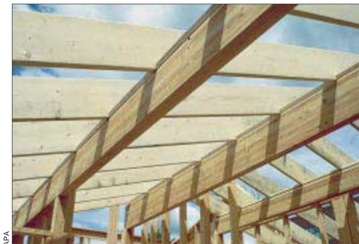
Figure 1. Use Architectural or Premium Grade glulams for exposed beams (left), and less expensive Industrial Grade for concealed beams (right).
