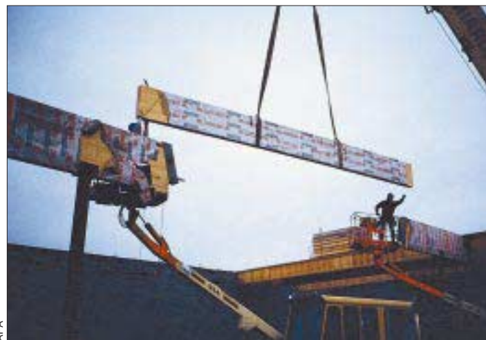
Figure 2. Unless your delivery truck has a boom, you'll need a crane to unload and place large glulams. Use slings to protect the beams.
