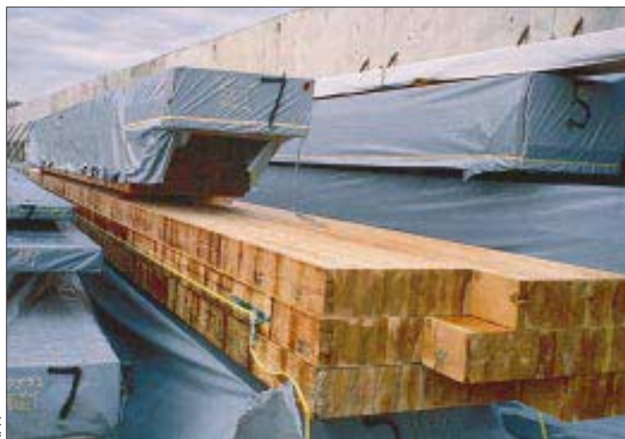
Figure 3. Glulams come to the job site wrapped in protective paper. To prevent uneven weathering and stains, it's best to unwrap the whole beam at one time.
