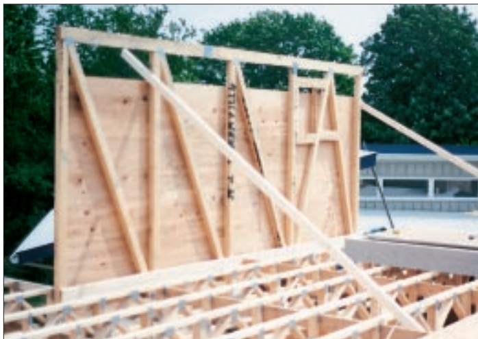
Built like an oversized truss sheathed with plywood, this girder wall carries roof loads from a 6-foot overhang down to the steel girder below.
