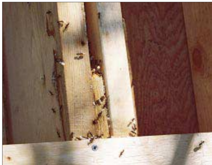
Figure 4. High moisture in the cathedral roofs created a perfect environment for carpenter ants, which tunneled into the insulation and nested in cracks between framing members.
