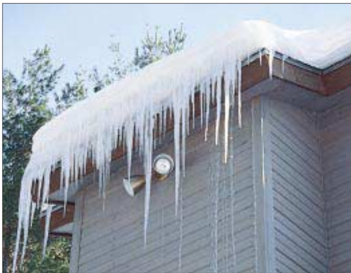
Figure 3. The winter before repairs were made, huge ice dams formed at the eaves of this cathedral roof. Water backed up into the soffits and walls, soaking interior and exterior finish materials.
