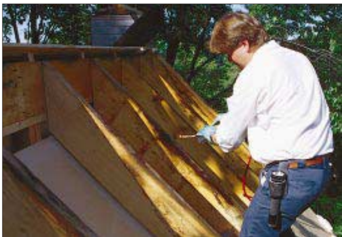
Figure 5. Before installing sister rafters and insulation, the existing framing was sprayed with a fungicide and insecticide.
