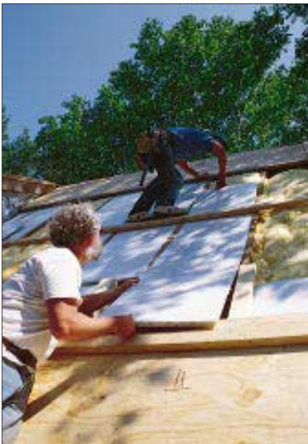
Figure 7. Two-by-four sleepers on top of existing rafters provide a ventilation chute beneath the plywood sheathing, while 1-inch rigid foam insulation prevents the fiberglass batts from expanding into the air space.
