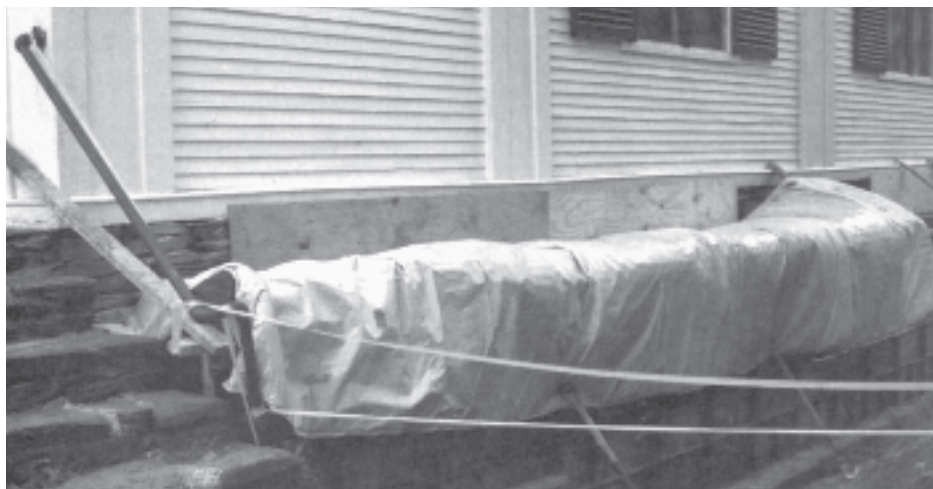
Figure 2. The most common way to protect freshly poured concrete is with insulation blankets. Make sure the edges of the blankets are weighted down to prevent convection currents.
