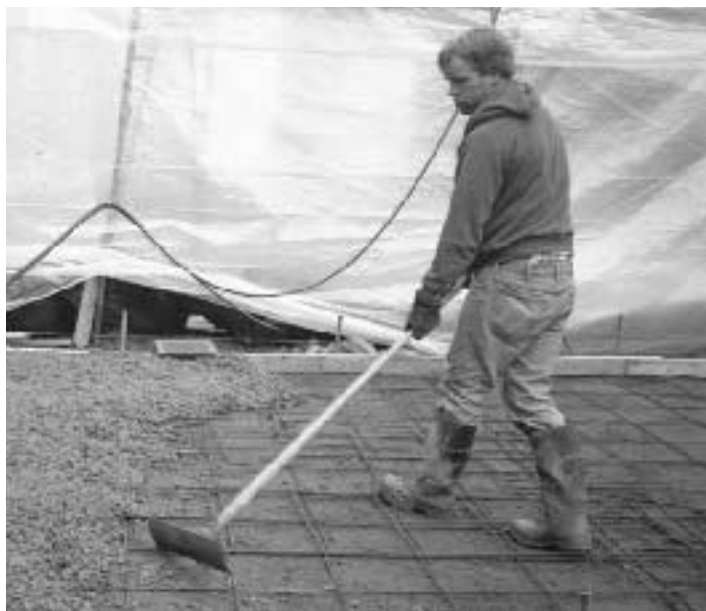
Figure 4. A heated enclosure made of wood and poly can be used to keep concrete at the ideal 55°F temperature.
