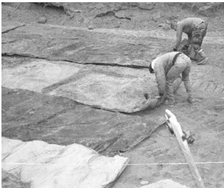
Figure 1. The subgrade must be thawed out before concrete is placed. If the frost is only a few inches deep, an insulating layer of straw (top) or an insulating blanket (bottom) will allow the earth's heat to thaw the ground.
